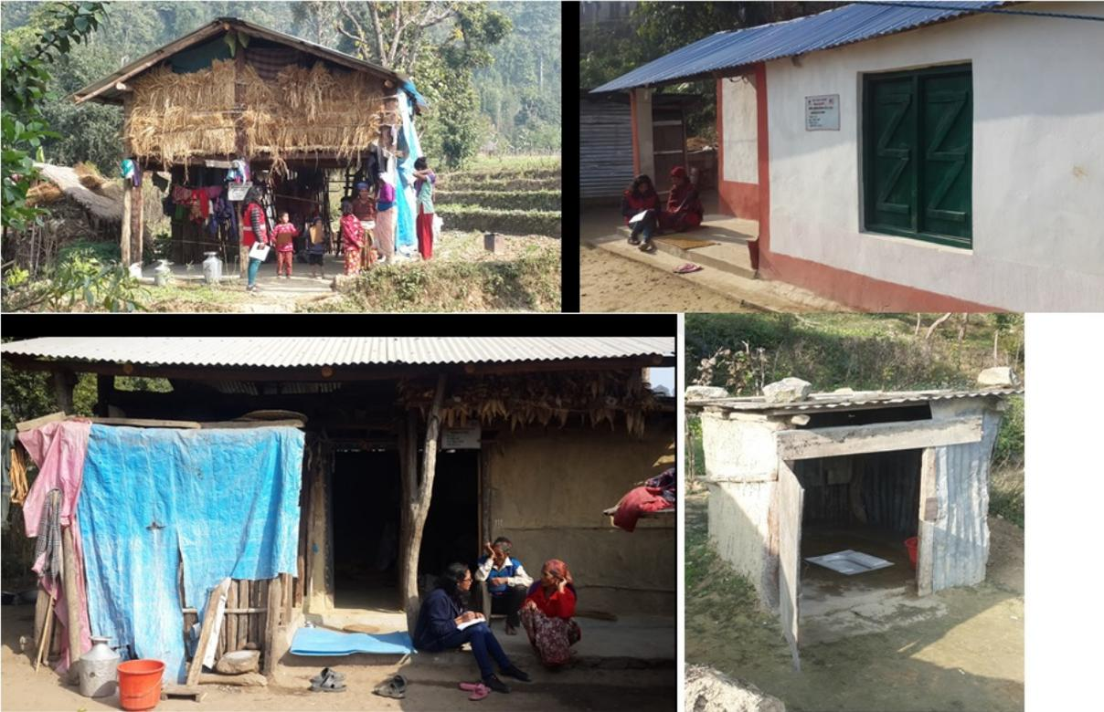
*The progressive shelter programme set basic criteria for construction (e.g. minimum two rooms, concrete floor covering specified foundation, latrine) but beneficiaries were responsible for construction and free to adapt design to their own needs and capacity to provide additional resources. The end results hence varied widely. The upper left picture shows the only house observed that had been constructed entirely within the NRS 60,000 subsidy.*
