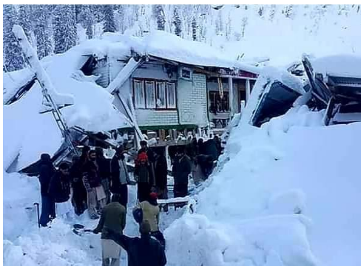
Houses damaged by heavy snowfall in Kashmir. (Photo source: PRCS)
