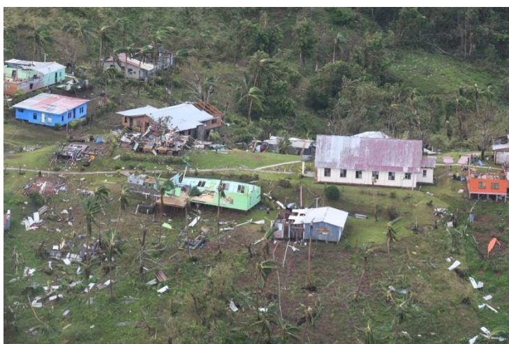
Aerial photo of damages in Vacalea village in Kadavu. (Photo: Fiji NDMO)
