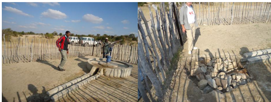
Functioning rehabilitated borehole with soak pit. Photo: IFRC
