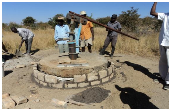
Water point in Mzimuni being rehabilitated. Borehole has not been working for the last 2 years and people were collecting water from a river 3 km away
