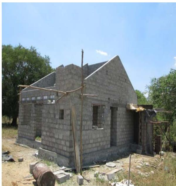
Figure 4 Adequate quality block work
