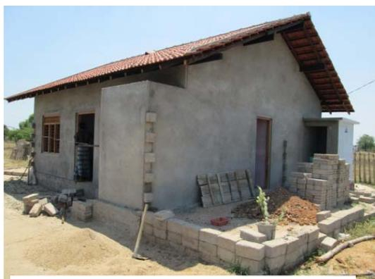
Figure 6 Gable roof and provision for future extensions
