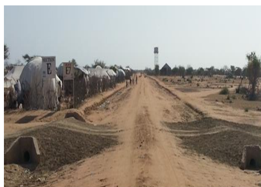
Completed works of the drainage system. Photo/ KRCS.
