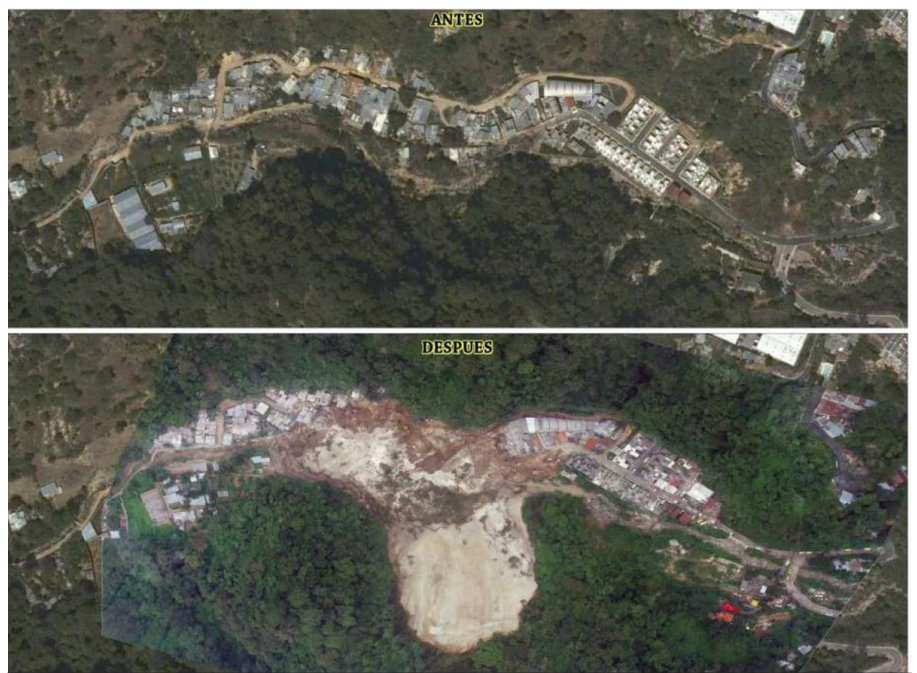
An aerial shot of before and after the landslide. Source: CONRED
