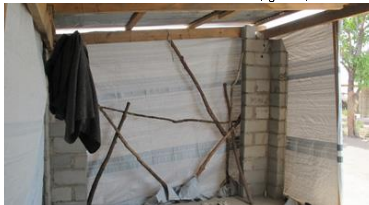
Some beneficiaries use sticks and tarps to make walls and they are exposed to be blown away by winds. Photo by IFRC
