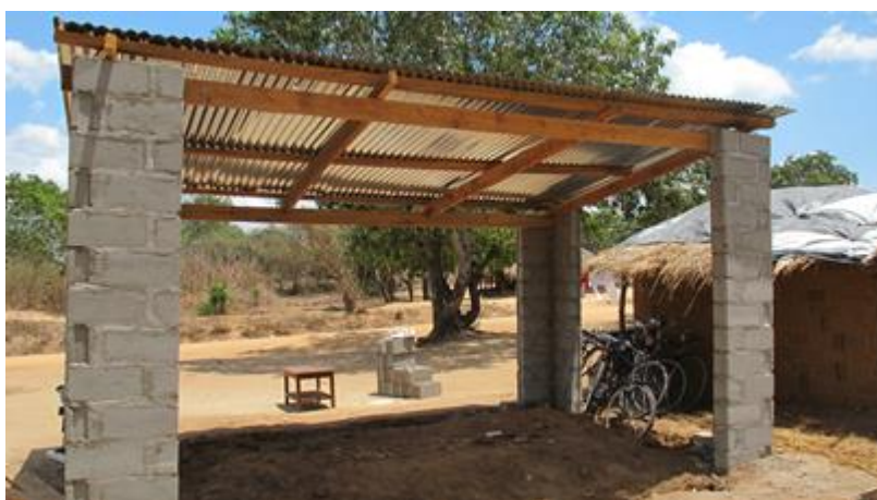
Delay in cement delivery leads to incompleteness of floor. Photo by IFRC
