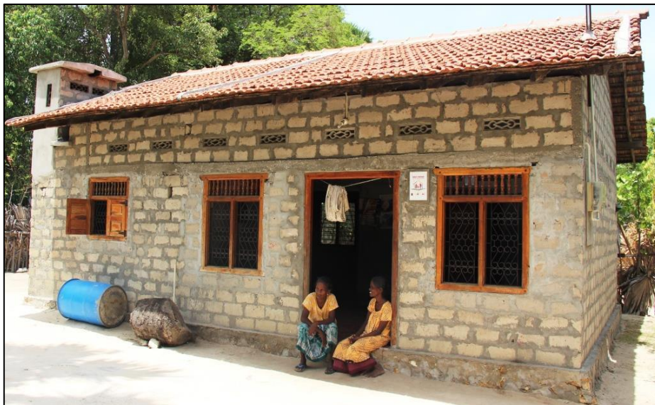
The recently completed new house of Ms. S. Poovathi; a beneficiary in Karainager, Jaffna. Photo: IFRC
