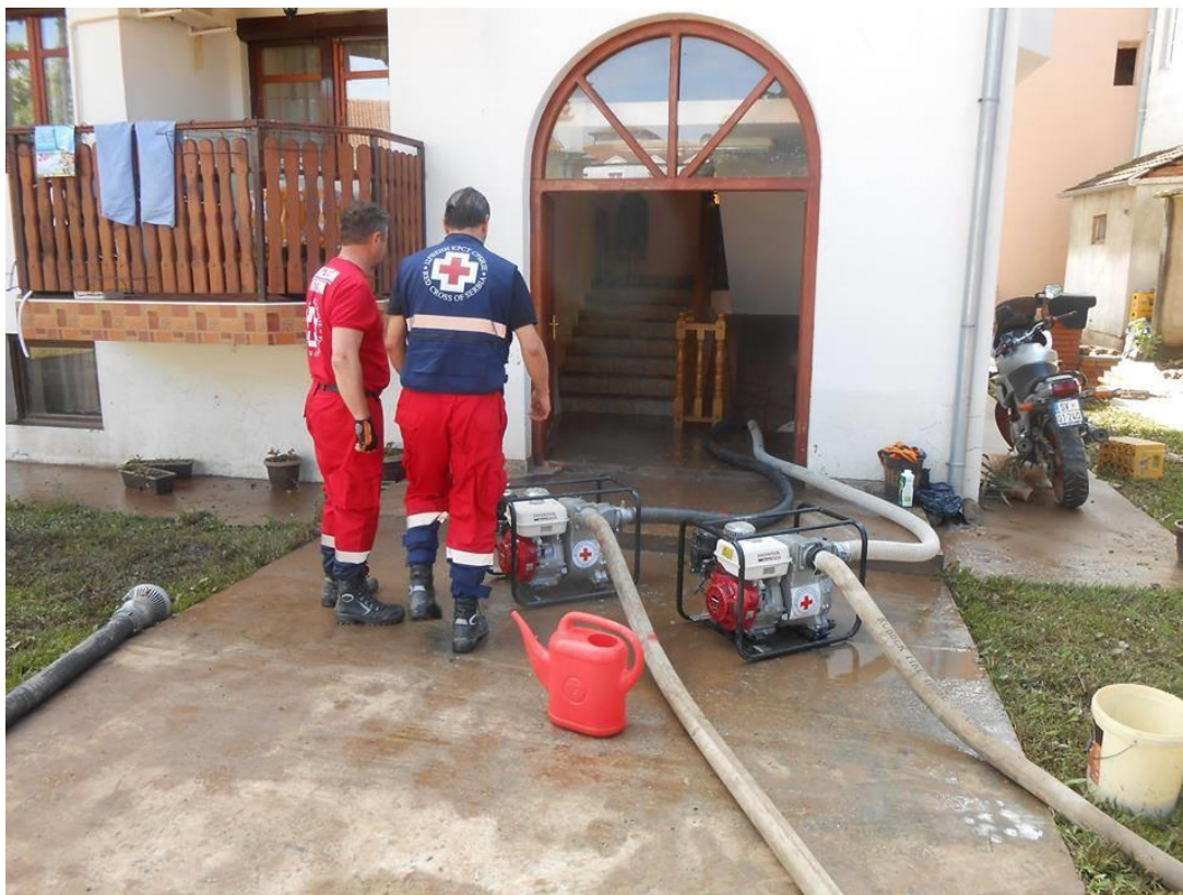
Mobile technical teams pumping water out of the basement of a flooded house. Photo: RC of Serbia
