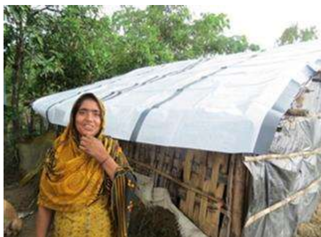
One of the beneficiaries standing next to her repaired house and expressing her appreciation for the tarpaulin given by BDRCS as part of the emergency shelter materials.
