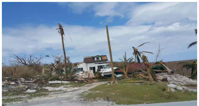
Damage to property, Long Island. Source: The Official Nassau Guardian (1844) Facebook
