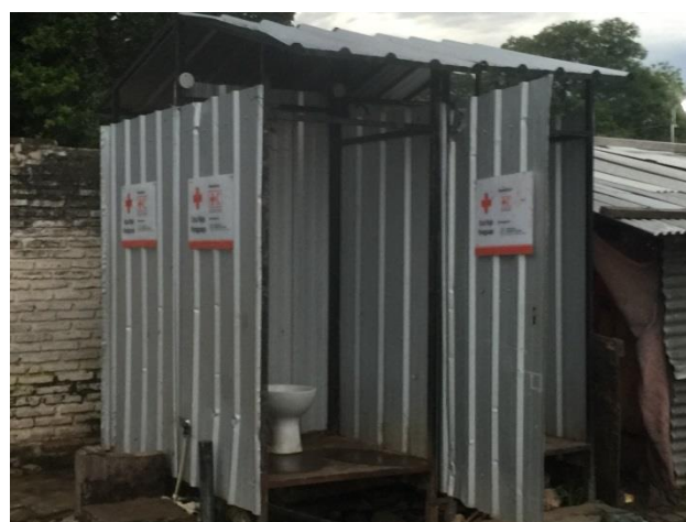
Installation of Paraguayan Red Cross sanitary modules in Asunción - Source: IFRC
