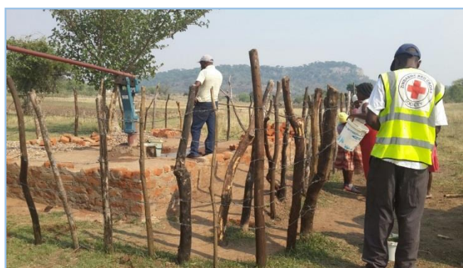
(b) Fenced borehole without apron and spillway
