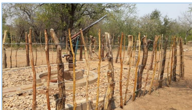
(a) Well fenced borehole with apron and spillway intact
