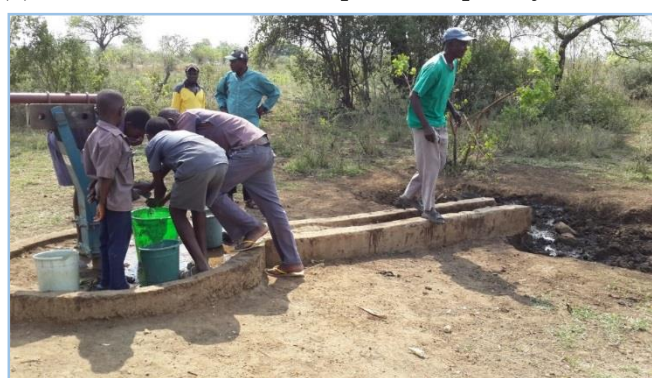
(d) Unfenced borehole with apron and spillway but with poor drainage
