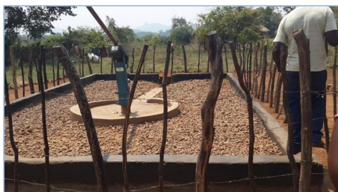
(c) Fenced borehole with complete apron and spillway
