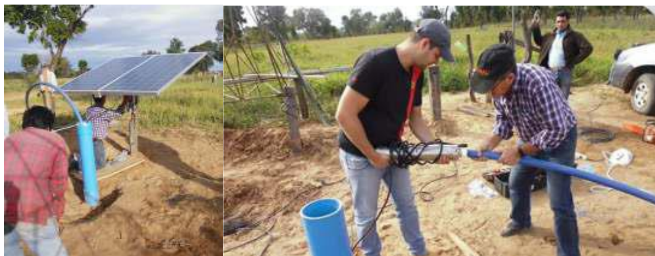
Work in the community of Jotoicha. Source: Paraguayan Red Cross.
