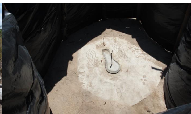
Concrete latrine slabs are in use in 1 de Maio.
