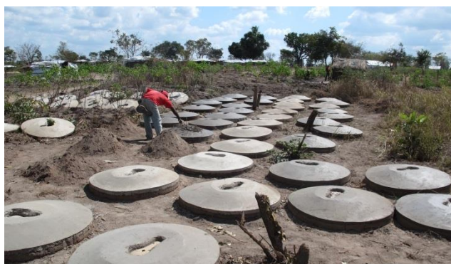
On site production of latrine slabs.
