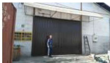
Photo 12: Refurbished warehouse of the RCSBiH in Sarajevo.
