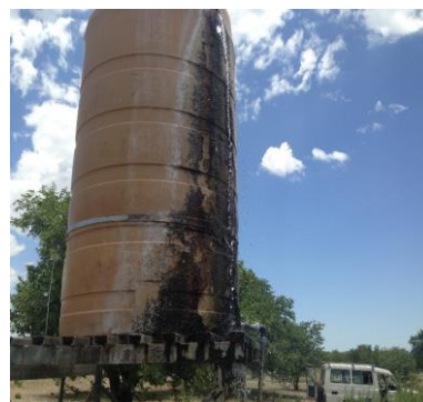
Community water tank for rehabilitation. Photo NRCS
