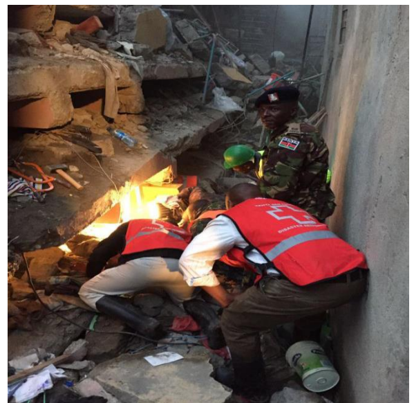
KRCS search and rescue teams continue to look for survivors in the collapse Huruma Estate building © KRCS
