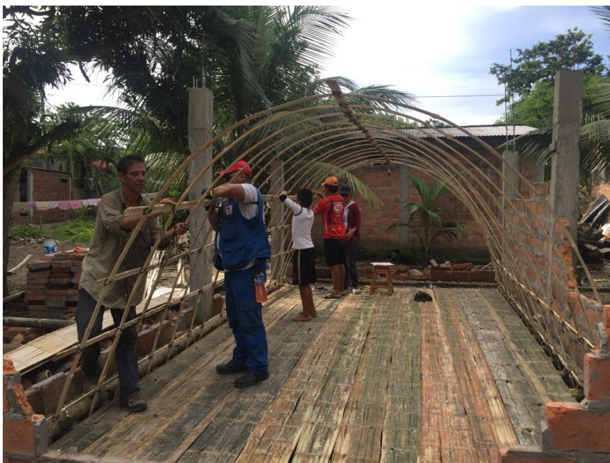
The ERC and IFRC using local materials have started teaching the affected population to build emergency shelters in Coaque, Manabí. Source: Spanish Red Cross
