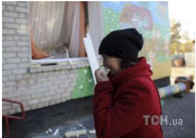
A destroyed home in Svatovo. By courtesy of TCH.ua
