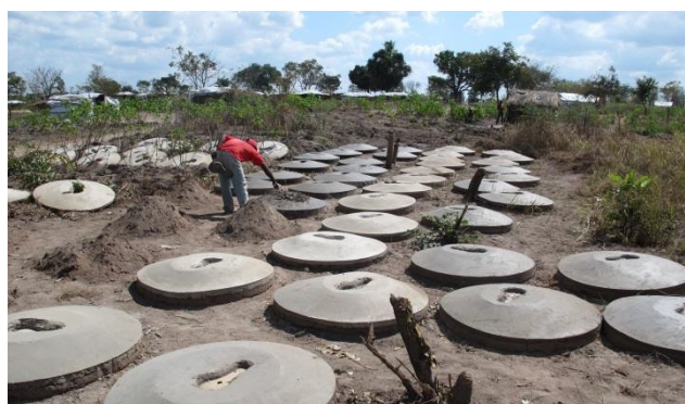
On site production of latrine slabs.
