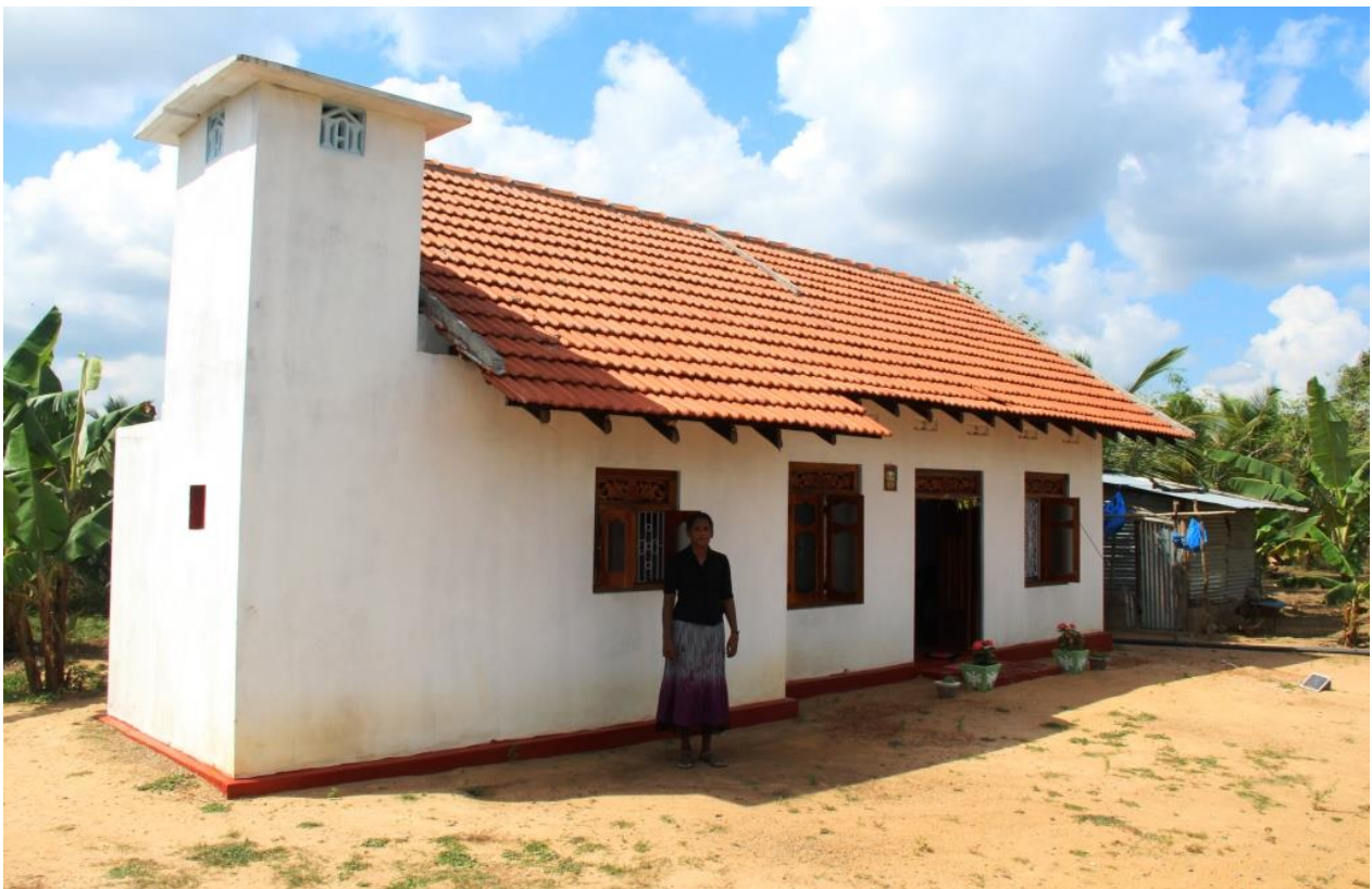
A beneficiary, who received assistance under RC PCRP to build a decent shelter through owner driven approach with more space and freedom had transformed lives of the families.
