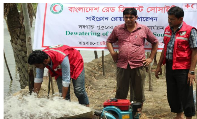
Dewatering of pond where saline water intrusion polluted the water, Photo Credit: BDRCS
