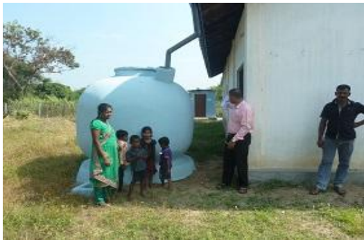
New Toilets and Repaired Rain Water Harvesting Facility funded by the IFRC in IHP area
