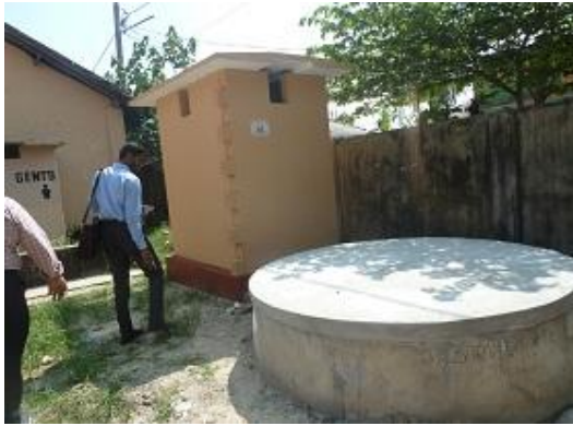
New Toilet Facility of a School funded by IFRC in IHP area
