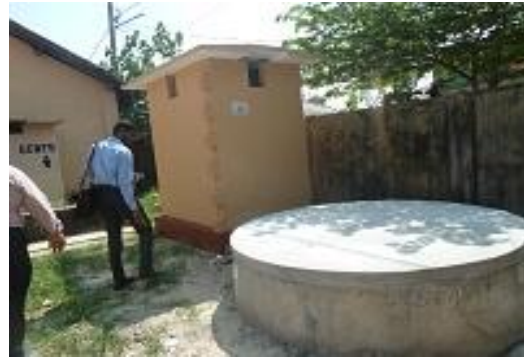
Sample of a single unit school toilet
