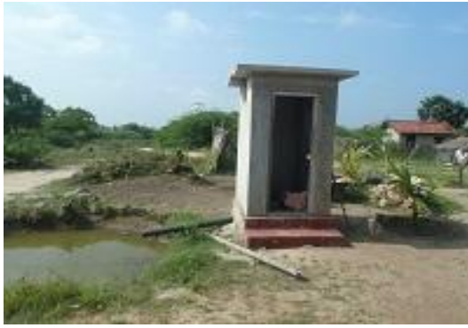
Toilet pit construction delayed due to high ground water table.(Rasapuram, Nanattan DS)
