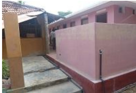
Sample school toilet complex-Puttur, Kopay DS
