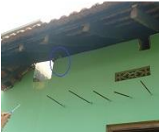
Roof components properly treated by preservatives, connected well and properly anchored
