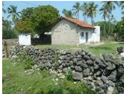
New toilet not constructed. Household using existing toilet. (Delft)
