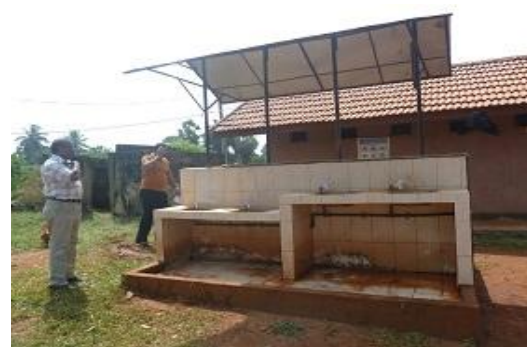
Repaired Water Facility funded by IFRC in IHP area
