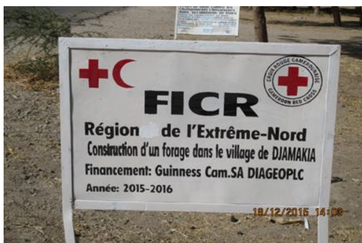
Visibility plate at borehole construction site in Djamakia © CRC
