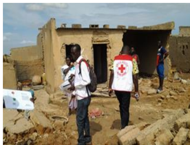
House damages caused by rains in Ouagadougou © BFRC
