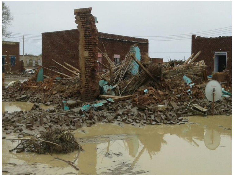
The recent floods damaged or destroyed over 10,474 homes across thirteen states of Sudan. Photo by SRCS Sennar Branch
