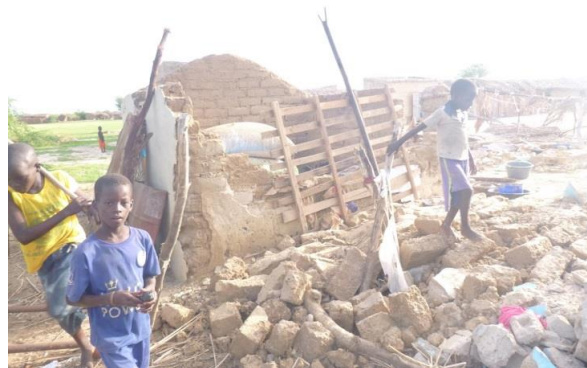
Houses destroyed after the heavy rains in Dagana. Photo /SRC
