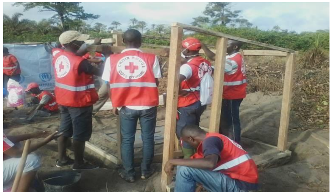
NDRT putting into practice construction of latrines in an emergency
