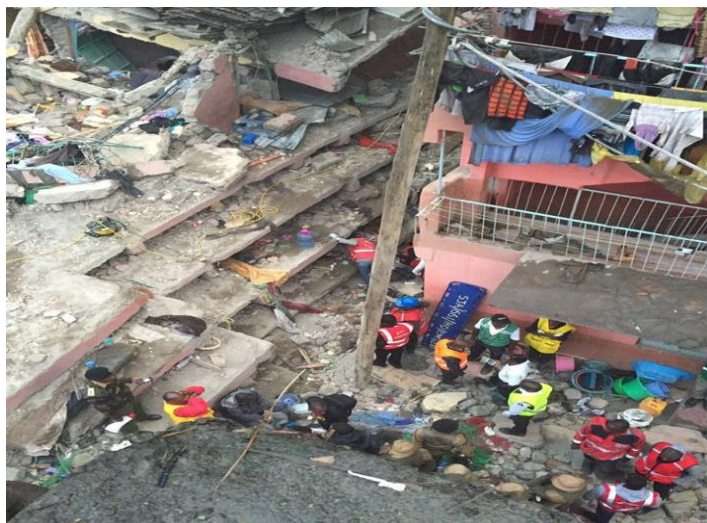
Figure 1: 'Pancake collapsed building'. Photo. KRCS
