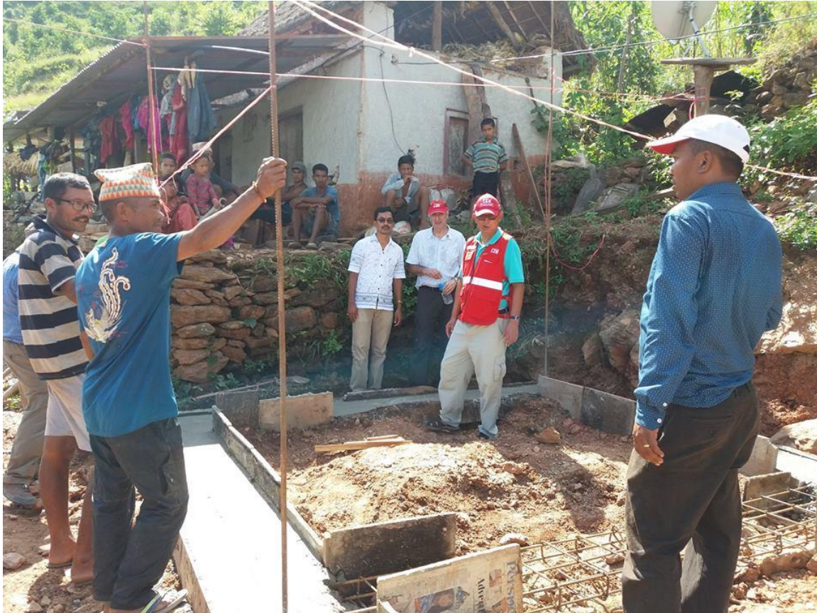
Shelter construction works have commenced in Sindhuli district, (Photo: NRCS)
