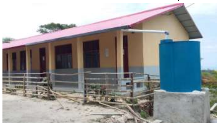
Water catchment and tank installed in school in Parlimento, (Photo: CVTL)
