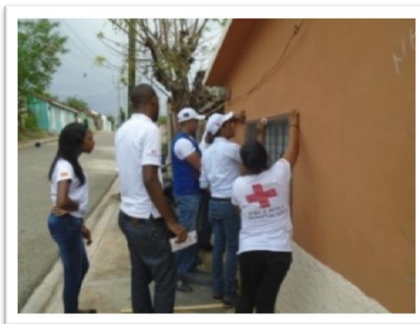
Volunteers installing wire mesh in targeted communities - Source: DRC
