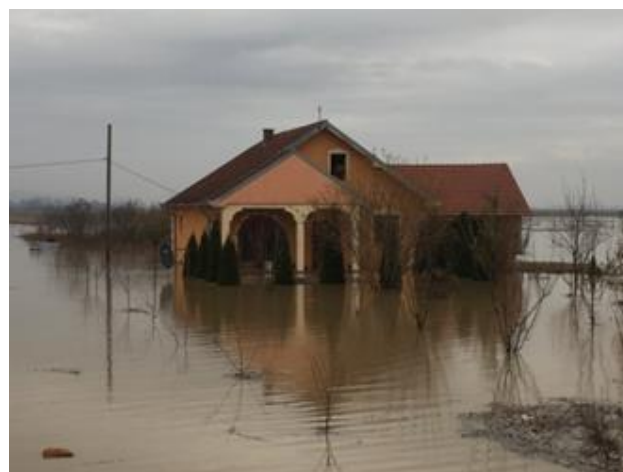
Flooded house in Kosovo*. Photo: RCSK
