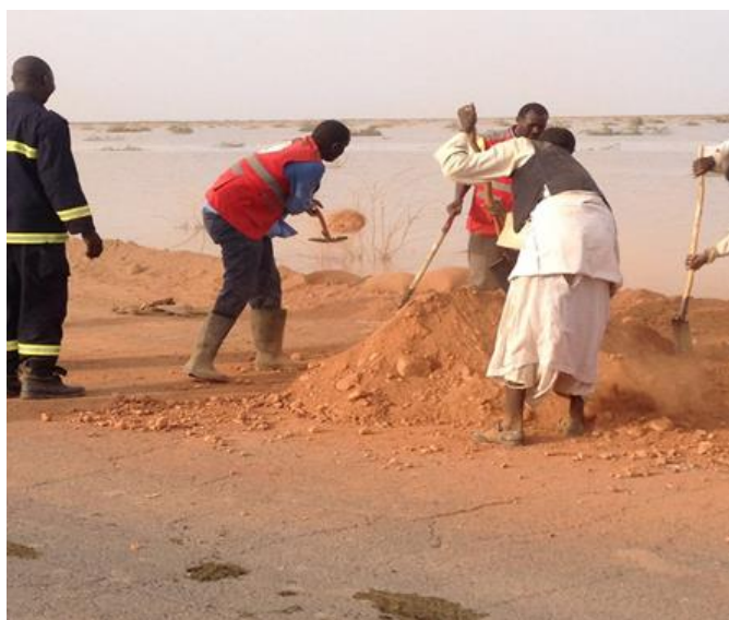
SRCS Volunteers building dykes. Photo SRCS
