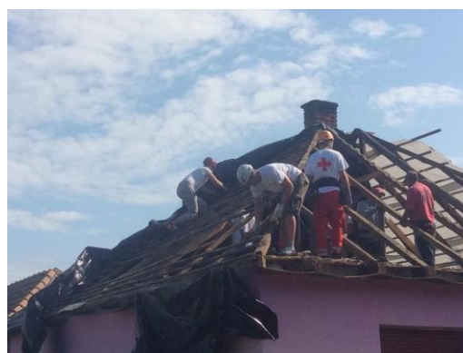
Repairs in progress in the affected area. Photo: HRC
