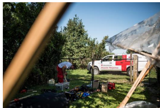
Repairs in progress in the affected area. Photo: HRC
