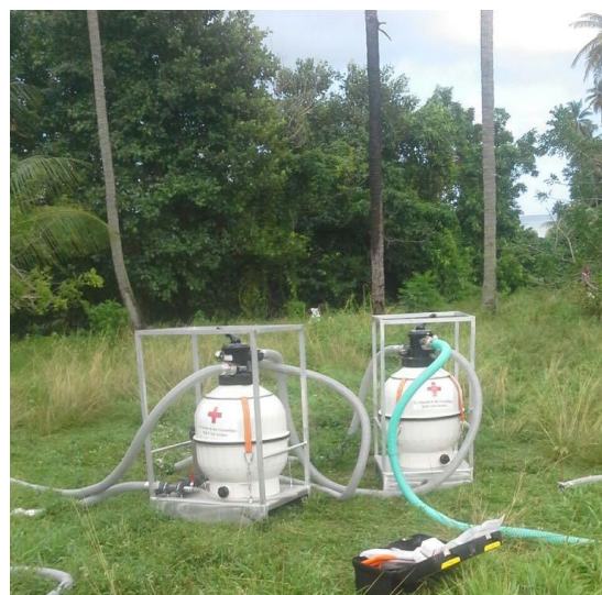
Water Plant in Georgetown Source: SVGRC
