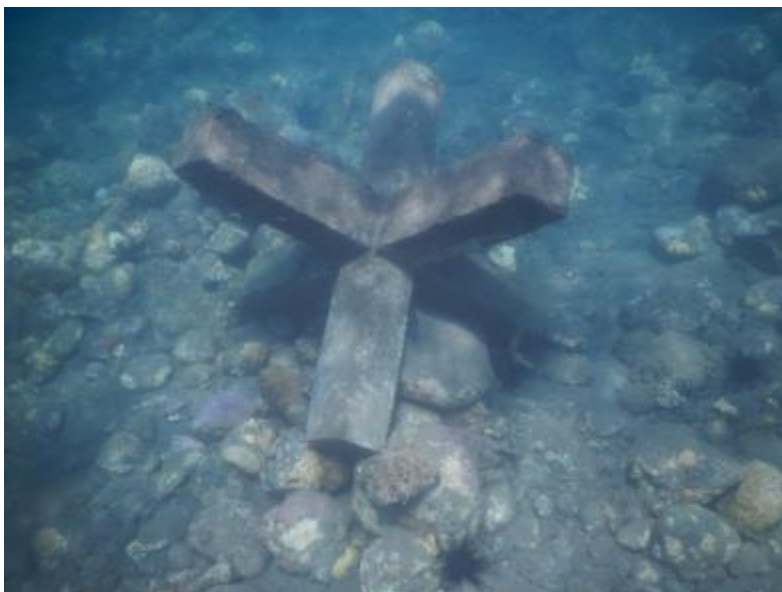
Concrete blocks were submerged within the marine sanctuary in Antique. This blocks would serve as temporary shelter for marine life while corals are still recovering to grow. Photo: Maryjoy Evalarosa/IFRC
