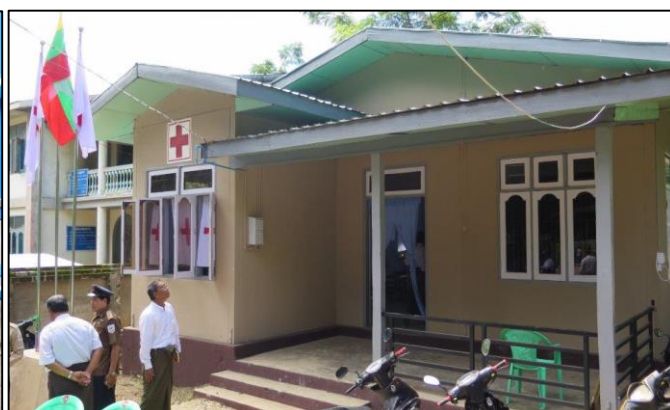
After MRCS' Tamu Branch building was damaged during the floods, it was renovated and reopened for use. (Photo: IFRC)
