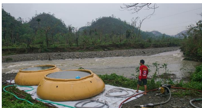
Two onion water bladder tanks have been setup in Virac, Catanduanes. Each onion bladder tank can store up to 10,000 L of water. Photo by Linus Escandor II/IFRC
