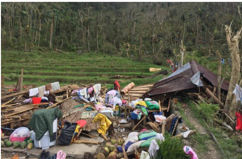
A damaged shelter in Bato municipality, Catanduanes. Thousands of homes were damaged in the island province of Catanduanes. Photo: PRC
