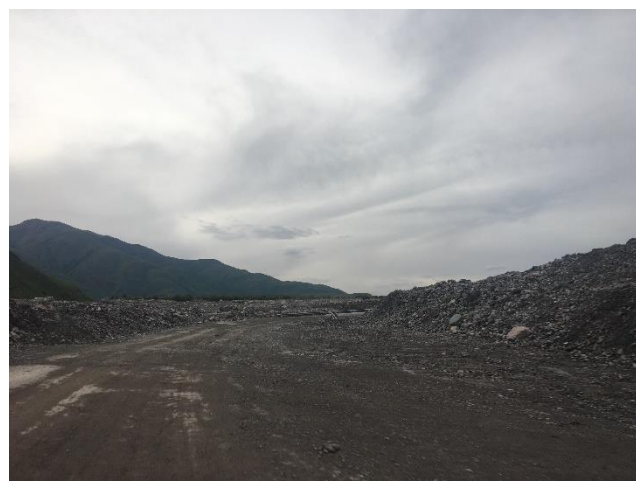
National Route 9: The road is completely blocked, preventing northbound travel from Volcán. Source: ARC
