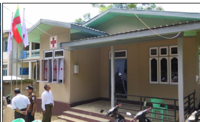
After MRCS' Tamu Branch building was damaged during the floods, it was renovated and reopened for use. (Photo: IFRC)
