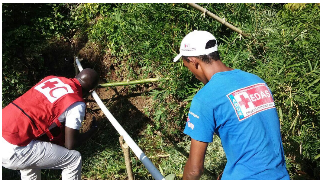
Photo 1: HRCS volunteers and WASH FACT member fixing the water distribution system at Anse d'Hainaut. Source: IFRC
