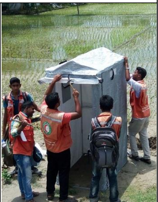
Volunteers installing mobile rapid latrine, (Photo: BDRCS)
