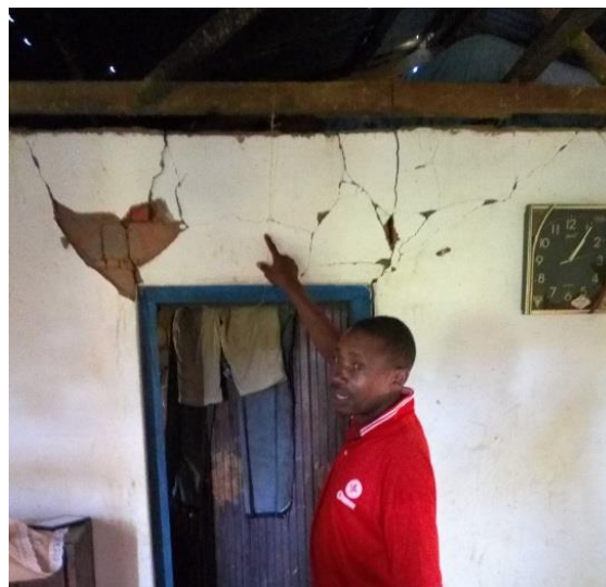
TRCS volunteers pointing the damage caused due to the earthquake. Photo: IFRC
