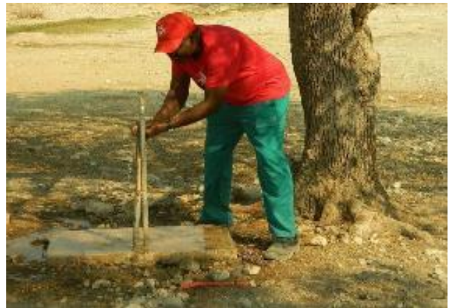
Community spring rehabilitated coupled with a water tap.
