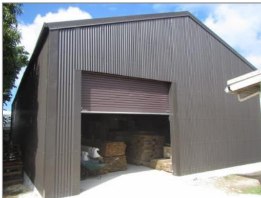
A new VRCS warehouse has been completed in mid-August 2016 and has been immediately put to use to store NFIs and construction materials for the WASH programme. A second warehouse is under construction for the VRCS branch office in Luganville, Santo Island. Photo: Francisco Fong/IFRC.
