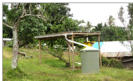
Rainwater collection system built in Sasake community, Emae. Photo: New Zealand Red Cross
