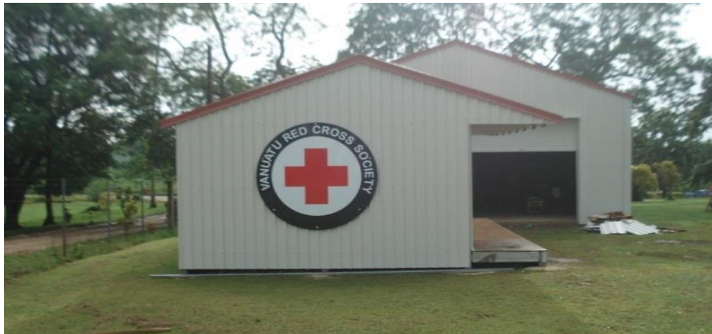
Both Santo Warehouse and annex building 100% completed: February 2016, (Photo: IFRC)
