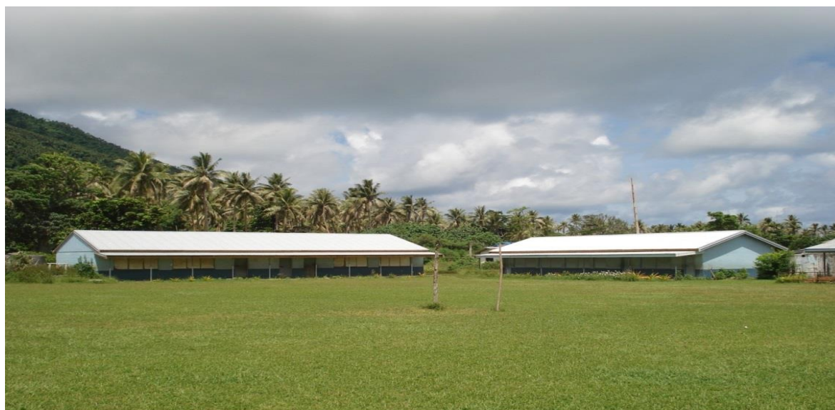
The picture above shows the two buildings in Nofo school that are rehabilitated by replacing the existing roofs and support structures. Photo: IFRC
