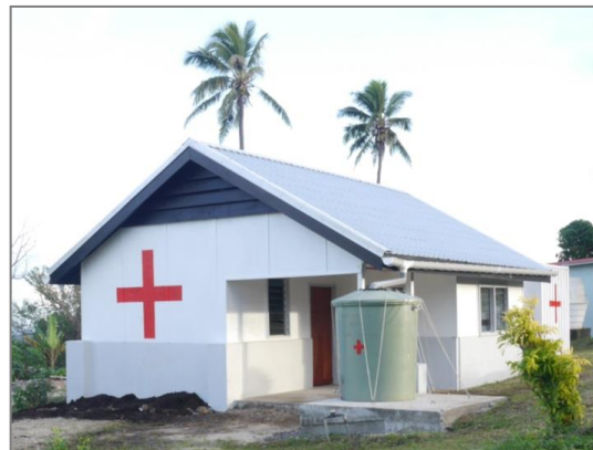
The VRCS Tafea branch office was completed in July 2016. IFRC and VRCS are currently building an annex to the building and will be used as additional office space for the VRCS and French Red Cross team in West Tanna. The new annex is expected to be completed by November 2016. Photo: Robbie Dodds/ Australian Red Cross
