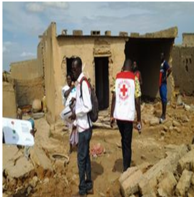
House damages caused by rains in Ouagadougou. BRCS/IFRC
