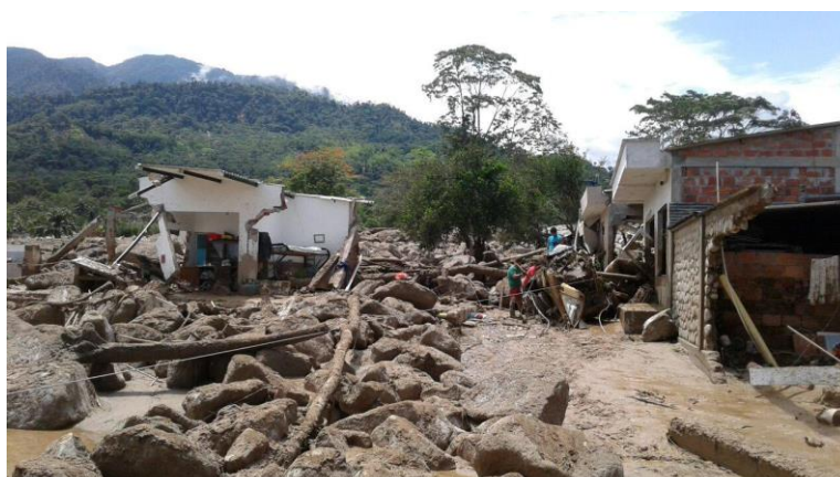
Damage to homes in the municipality of Mocoa in the department of Putumayo. Source: CRCS
